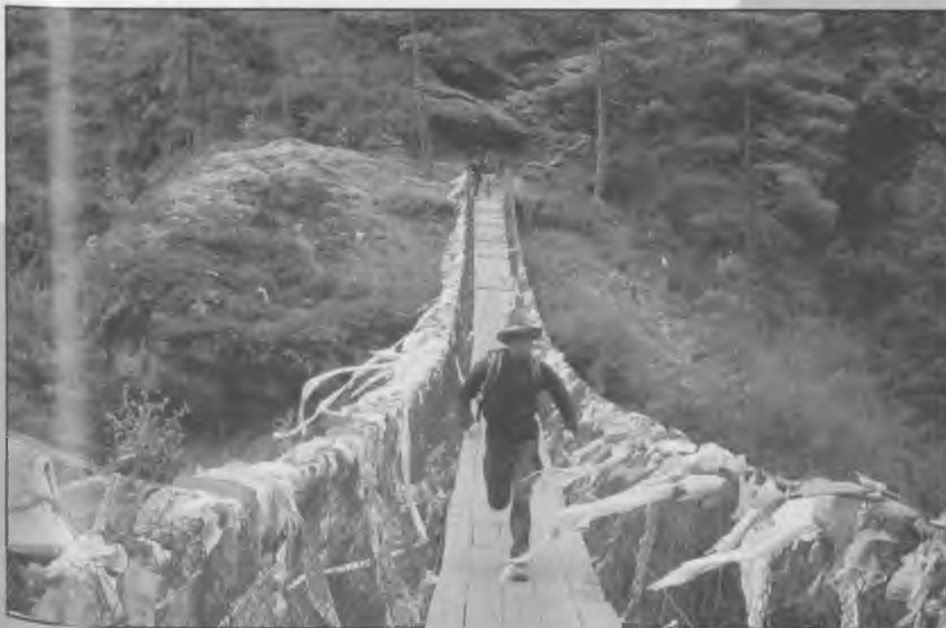
Adrian charges across the bridge at Tammy (Photo Neil Denby)
